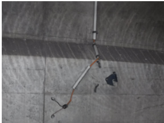
Emplacement de plot vide (arrachement)
